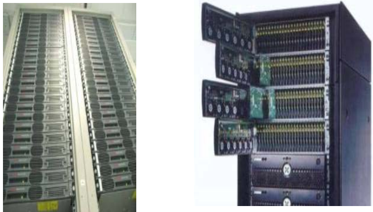
Figure 1 – Examples of compaction
